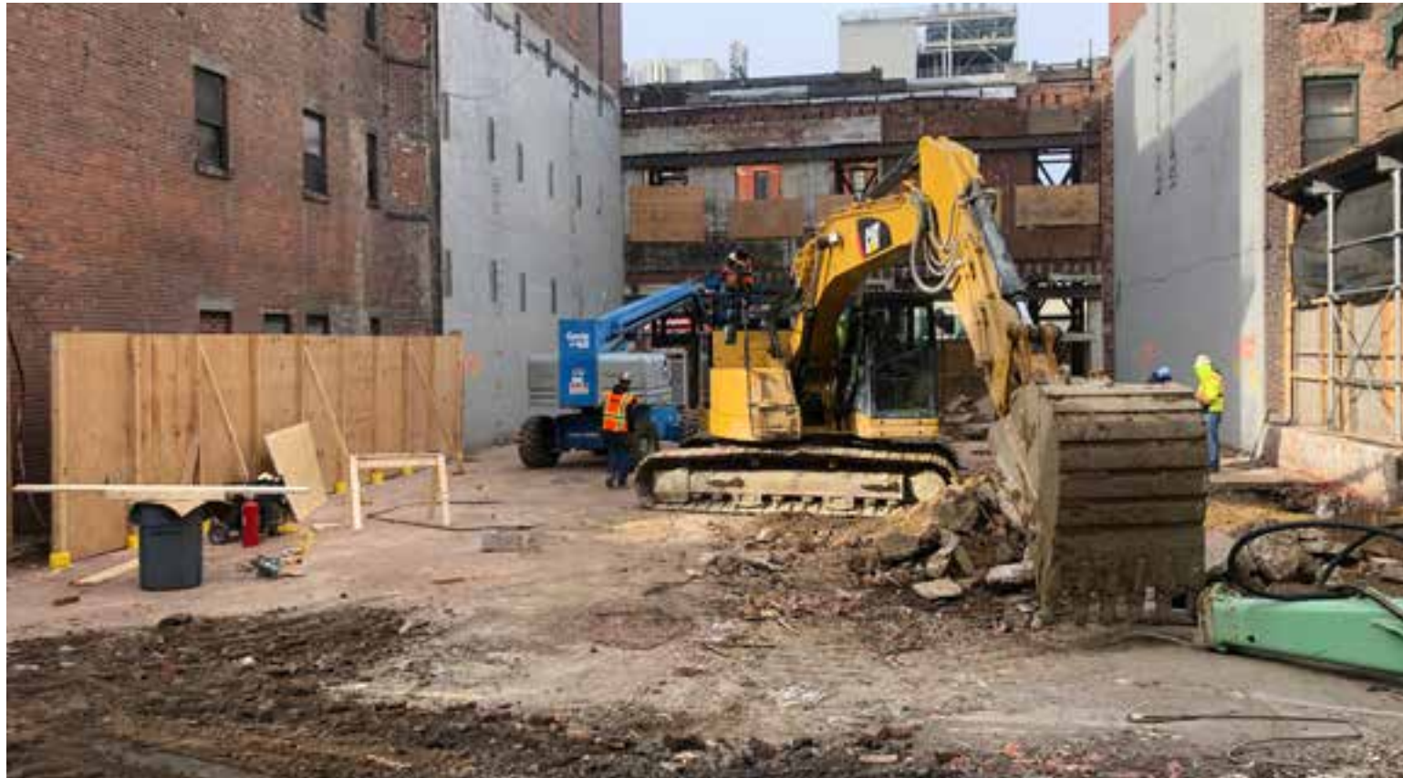
Ram hoes and back hoes brought on site to begin excavation
