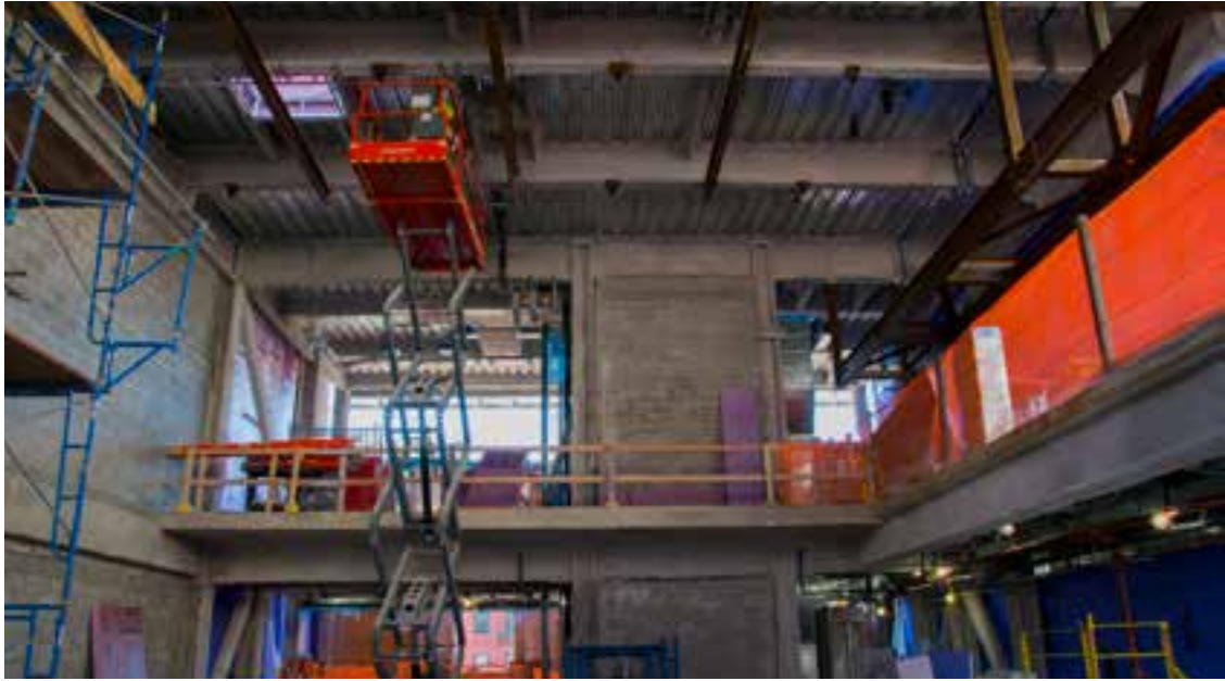
A scissor lift raises workers to install the beams and brackets for an advanced trolley system in our wire tension grid, allowing maximum mobility and flexibility for lighting and sound equipment
