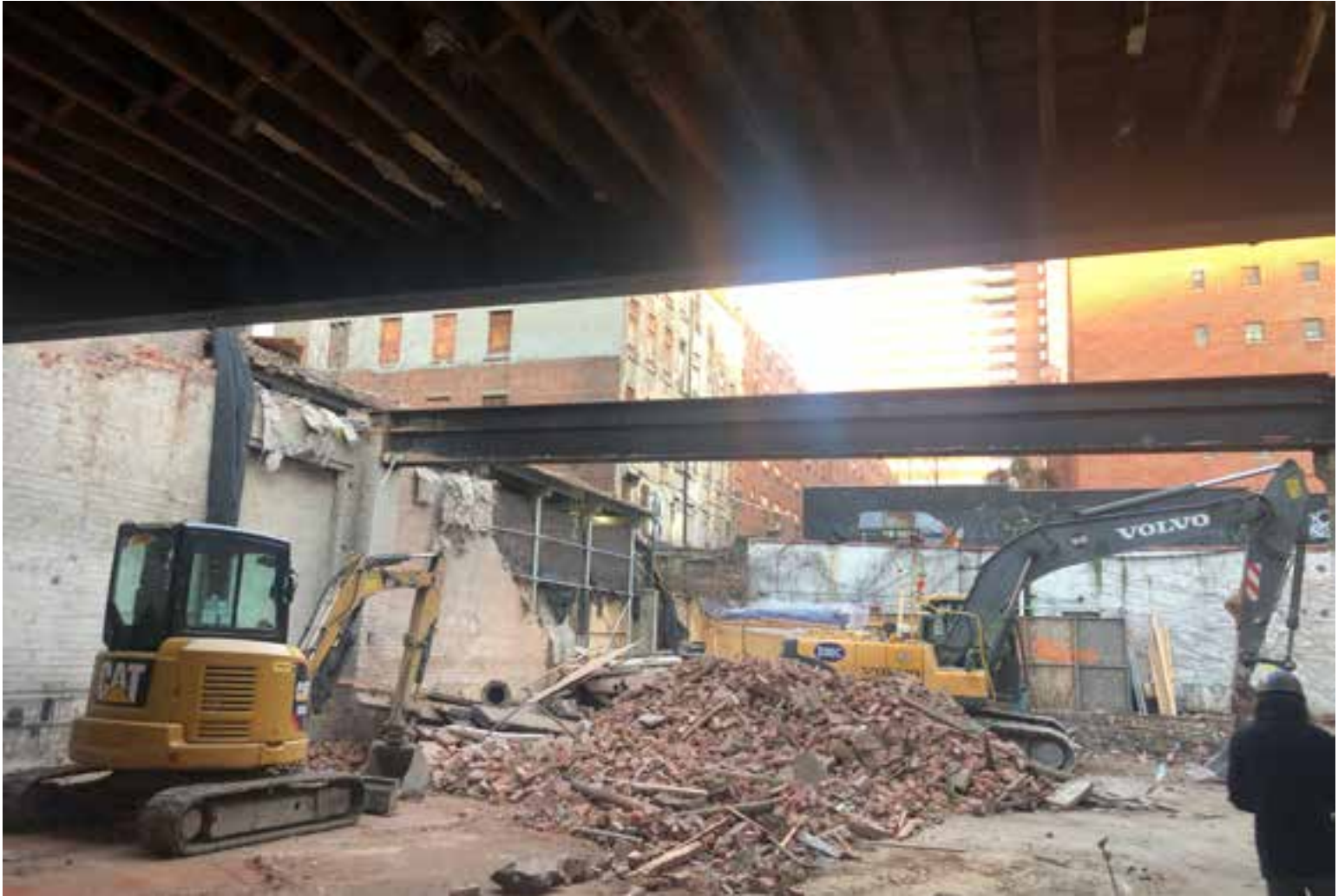
With rear wall demolition complete, the former Cybert Tire structure's steel girders remain, helping fortify the adjacent buildings during demolition
