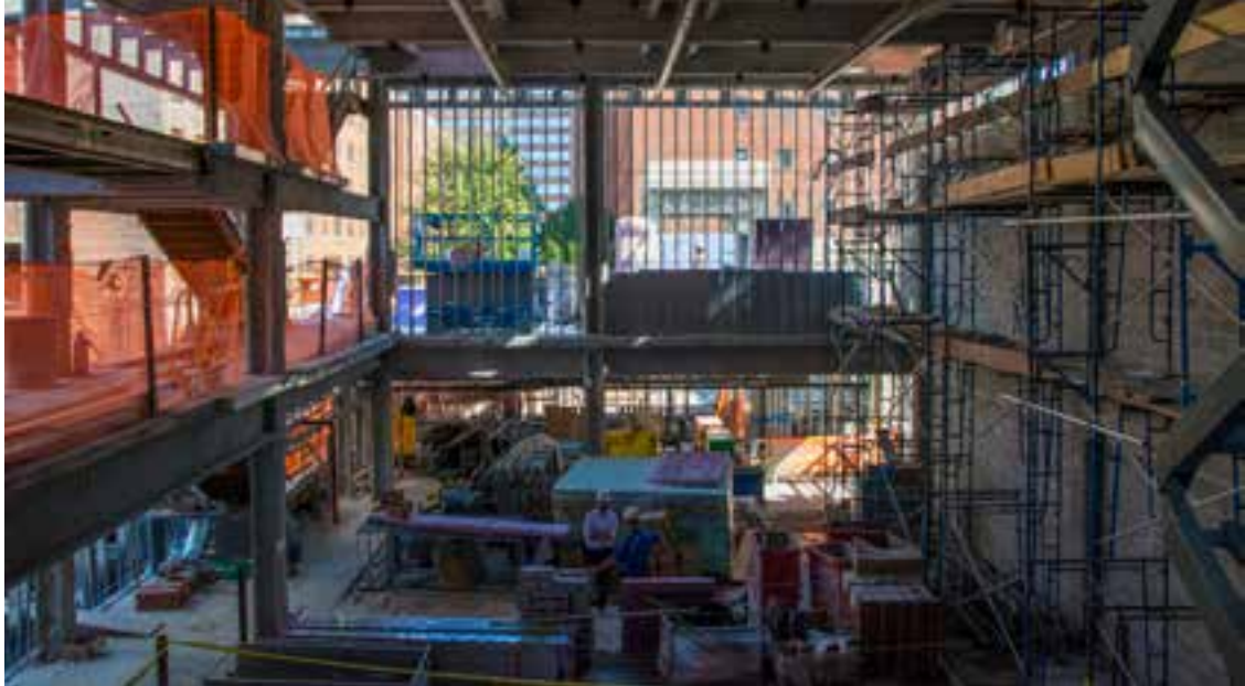
The walls are built for complete acoustic separation: a thick cinderblock, with each gap filled with concrete, with an additional layer of thick, dense, acoustically engineered sheetrock
